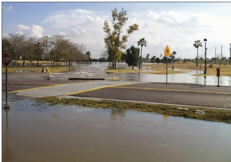
**Figure 2.** Indian Bend Wash, Scottsdale, Arizona, during a flood that covered a large portion of the “greenway”; the flood spread out over parks, golf courses, and streets, but resulted in minimal damage. This design was one of the first non-structural flood management systems in the US, created by local and federal government officials after damaging floods occurred in the 1960s.
